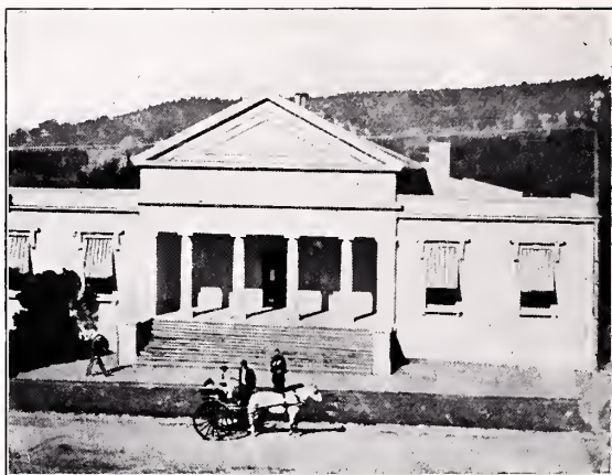
THE OLD COMMERCIAL HALL, GRAHAMSTOWN
